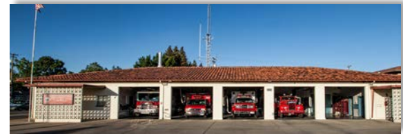
STATION #101 3000 Fulton Avenue Sacramento
