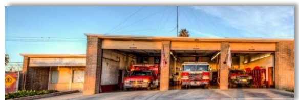
STATION #41 6900 Thomas Drive North Highlands
