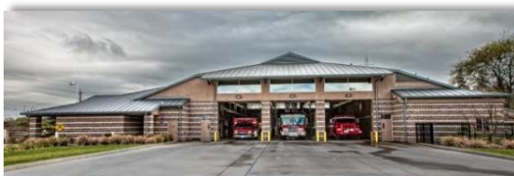
STATION #32 8890 Roediger Lane Fair Oaks
