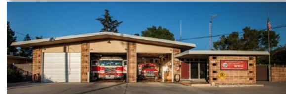
STATION #103 3824 Watt Avenue Sacramento
