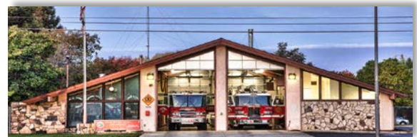
STATION #62 3646 Bradshaw Road Sacramento
