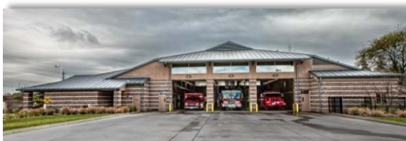
STATION #32 8890 Roediger Lane Fair Oaks
