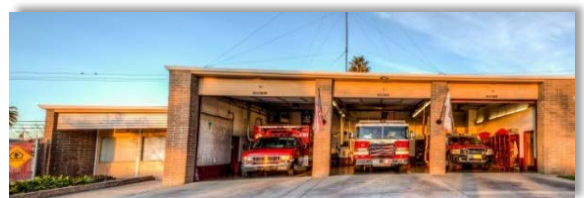
STATION #41 6900 Thomas Drive North Highlands
