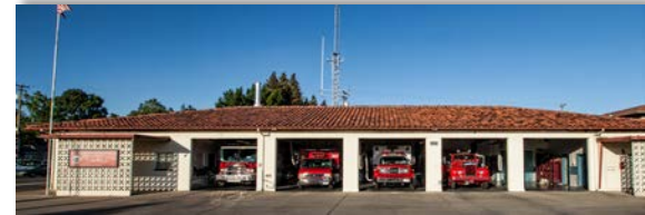
STATION #101 3000 Fulton Avenue Sacramento
