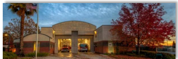
STATION #26 8000 Palmerson Drive Antelope
