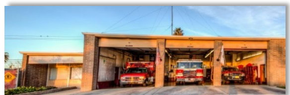
STATION #41 6900 Thomas Drive North Highlands
