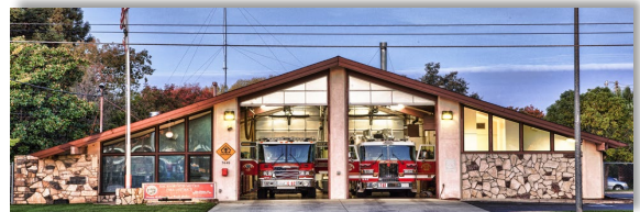
STATION #62 3646 Bradshaw Road Sacramento
