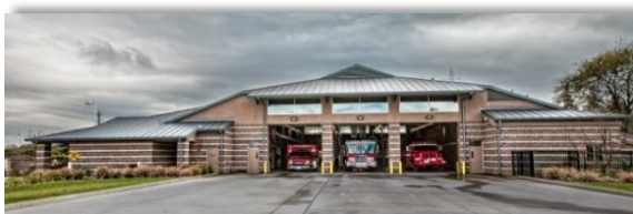
STATION #32 8890 Roediger Lane Fair Oaks
