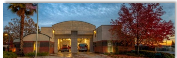
STATION #26 8000 Palmerson Drive Antelope
