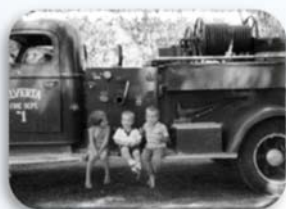
Elverta Fire District
