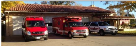
STATION #102 4501 Marconi Avenue Sacramento
