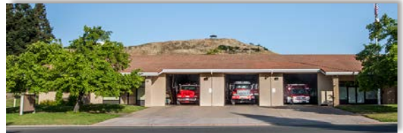
STATION #59 7210 Murieta Drive Rancho Murieta
