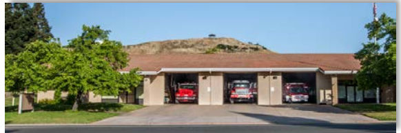
STATION #59 7210 Murieta Drive Rancho Murieta
