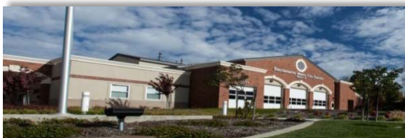
STATION #29 8681 Greenback Lane Orangevale
