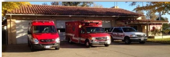
STATION #102 4501 Marconi Avenue Sacramento
