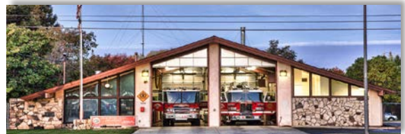
STATION #62 3646 Bradshaw Road Sacramento
