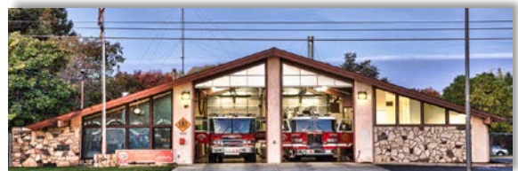
STATION #62 3646 Bradshaw Road Sacramento
