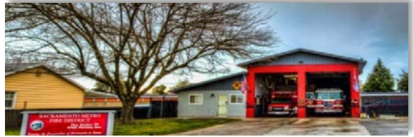
STATION #53 6722 Fleming Avenue Sacramento
