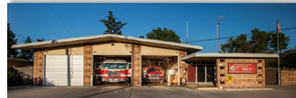
STATION #103 3824 Watt Avenue Sacramento
