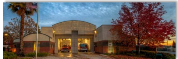
STATION #26 8000 Palmerson Drive Antelope
