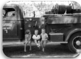
Elverta Fire District
