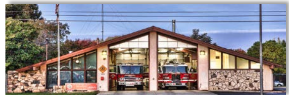
STATION #62 3646 Bradshaw Road Sacramento
