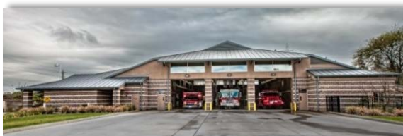
STATION #32 8890 Roediger Lane Fair Oaks
