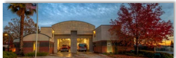
STATION #26 8000 Palmerson Drive Antelope
