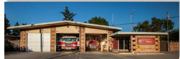
STATION #103 3824 Watt Avenue Sacramento
