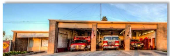
STATION #41 6900 Thomas Drive North Highlands
