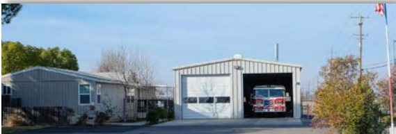
STATION #117 7961 Cherry Brook Drive Elverta
