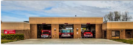
STATION #65 11201 Coloma Road Rancho Cordova
