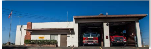
STATION #116 7995 Elwyn Avenue Elverta
