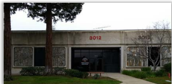
LOGISTICS/TRAINING/SAFETY 3012 Gold Canal Drive Rancho Cordova
