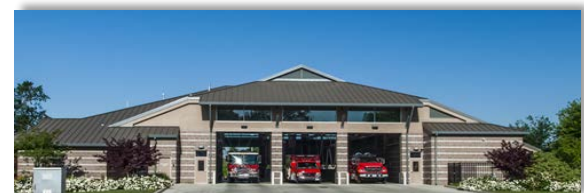
STATION #111 6609 Rio Linda Blvd. Rio Linda
