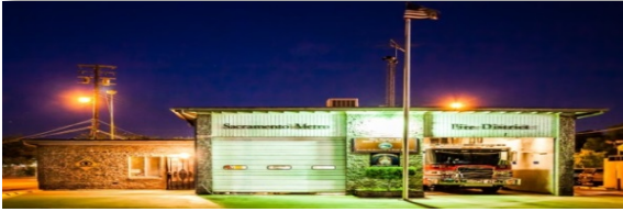
STATION #42 5608 North Haven North Highlands
