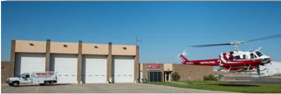
STATION #115 4727 Kilzer Avenue McClellan
