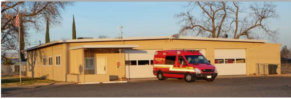
STATION #112 6801 34th Street North Highlands
