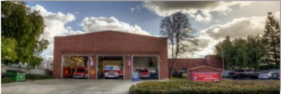
STATION #51 8210 Meadowhaven Drive Sacramento
