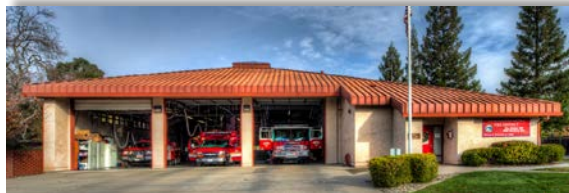
STATION #105 2691 Northrop Avenue Sacramento
