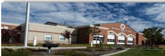
STATION #29 8681 Greenback Lane Orangevale
