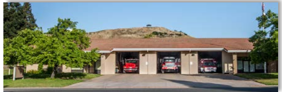
STATION #59 7210 Murieta Drive Rancho Murieta
