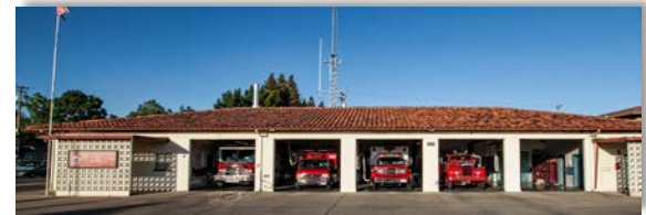
STATION #101 3000 Fulton Avenue Sacramento
