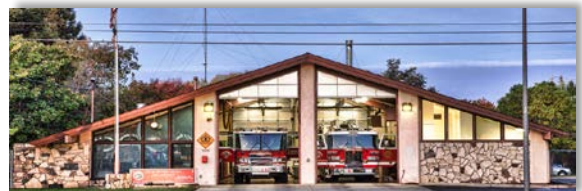
STATION #62 3646 Bradshaw Road Sacramento
