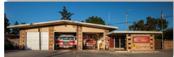
STATION #103 3824 Watt Avenue Sacramento
