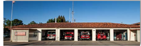
STATION #101 3000 Fulton Avenue Sacramento
