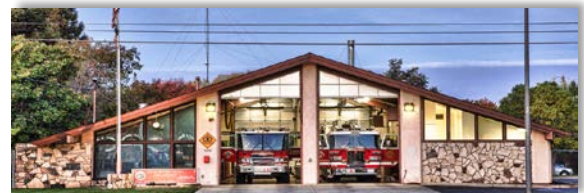
STATION #62 3646 Bradshaw Road Sacramento
