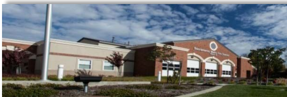
STATION #29 8681 Greenback Lane Orangevale
