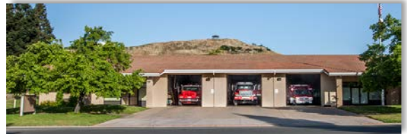
STATION #59 7210 Murieta Drive Rancho Murieta
