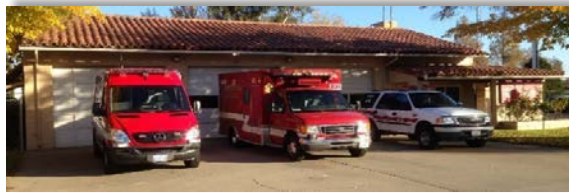
STATION #102 4501 Marconi Avenue Sacramento
