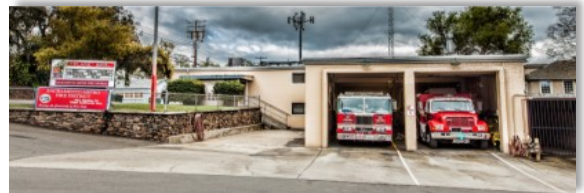
STATION #31 7950 California Avenue Fair Oaks
