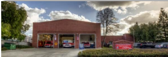
STATION #51 8210 Meadowhaven Drive Sacramento
