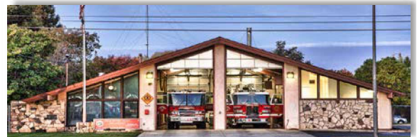
STATION #62 3646 Bradshaw Road Sacramento
