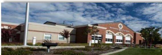
STATION #29 8681 Greenback Lane Orangevale
