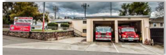
STATION #31 7950 California Avenue Fair Oaks
