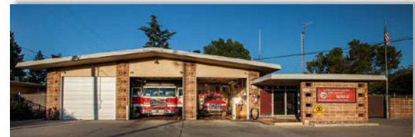
STATION #103 3824 Watt Avenue Sacramento
