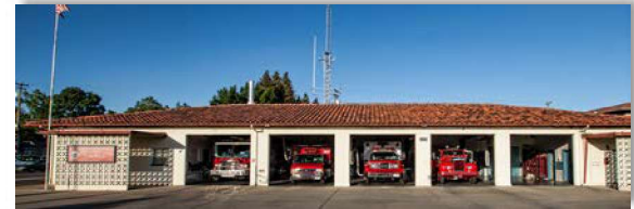
STATION #101 3000 Fulton Avenue Sacramento
