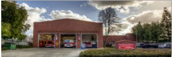
STATION #51 8210 Meadowhaven Drive Sacramento
