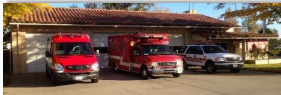
STATION #102 4501 Marconi Avenue Sacramento
