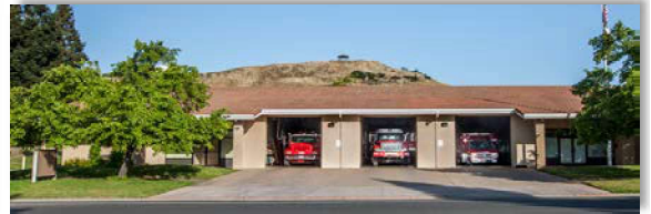
STATION #59 7210 Murieta Drive Rancho Murieta
