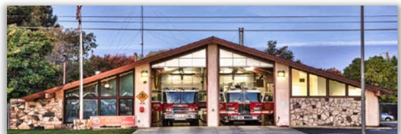
STATION #62 3646 Bradshaw Road Sacramento
