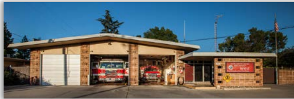
STATION #103 3824 Watt Avenue Sacramento
