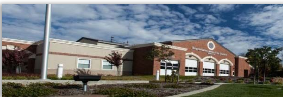
STATION #29 8681 Greenback Lane Orangevale
