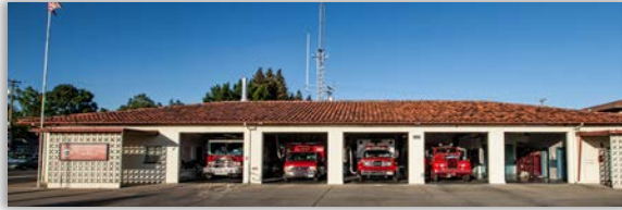
STATION #101 3000 Fulton Avenue Sacramento
