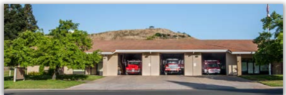
STATION #59 7210 Murieta Drive Rancho Murieta
